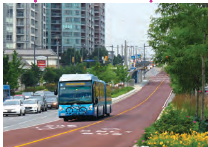
Highway 7 East rapidway, Richmond Hill and Markham
