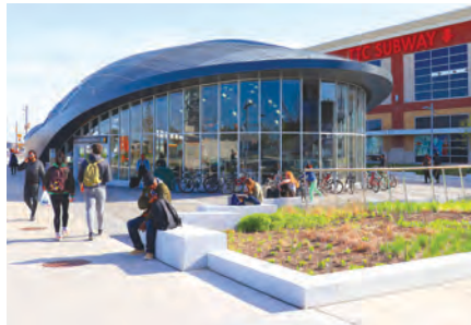
Toronto-York Spadina Subway Extension
