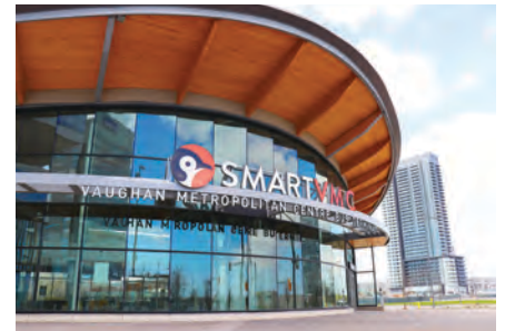
SmartVMC Bus Terminal
